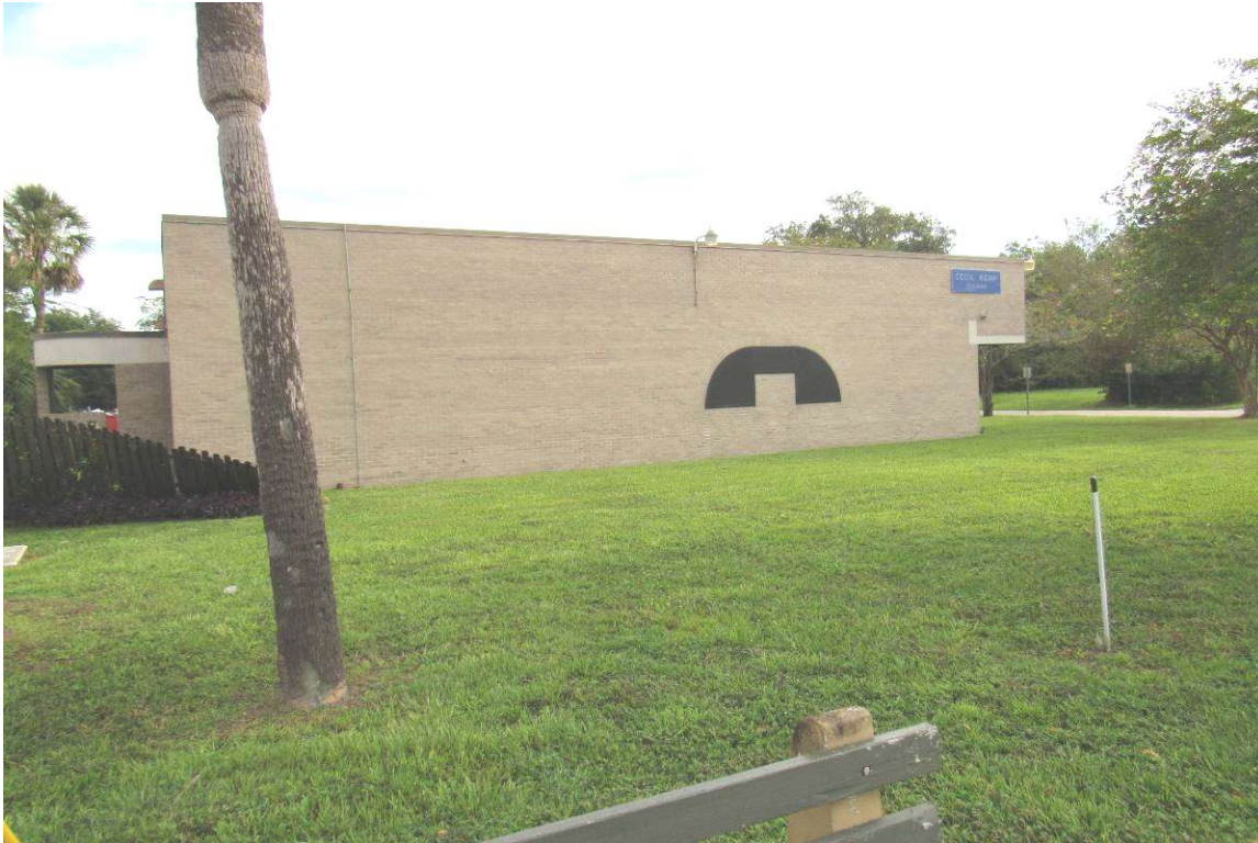
Existing State office building on subject property.
